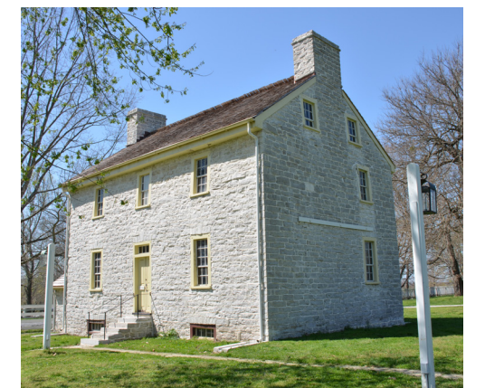
Cleaning and repointing success, 2020
